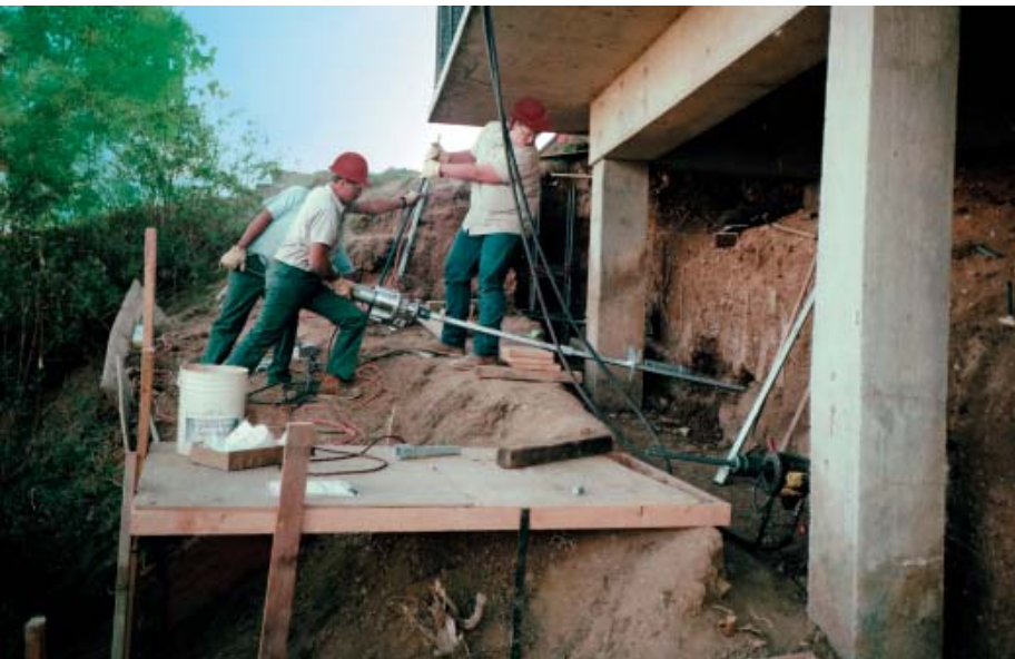
Chance® portable power-drive heads can get into most remote and limited-access work spaces.
