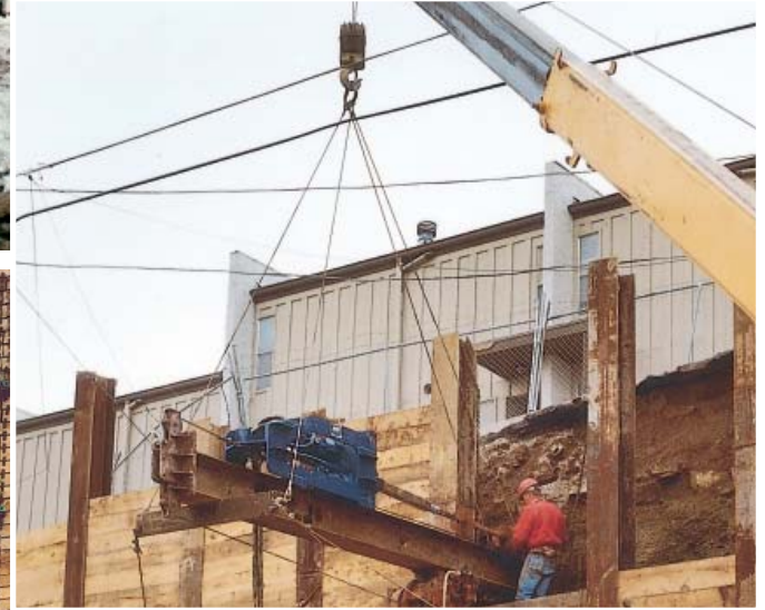
Lead-guided drill motors (crane-suspended or track-mounted) are common tieback drive equipment for large jobs.
