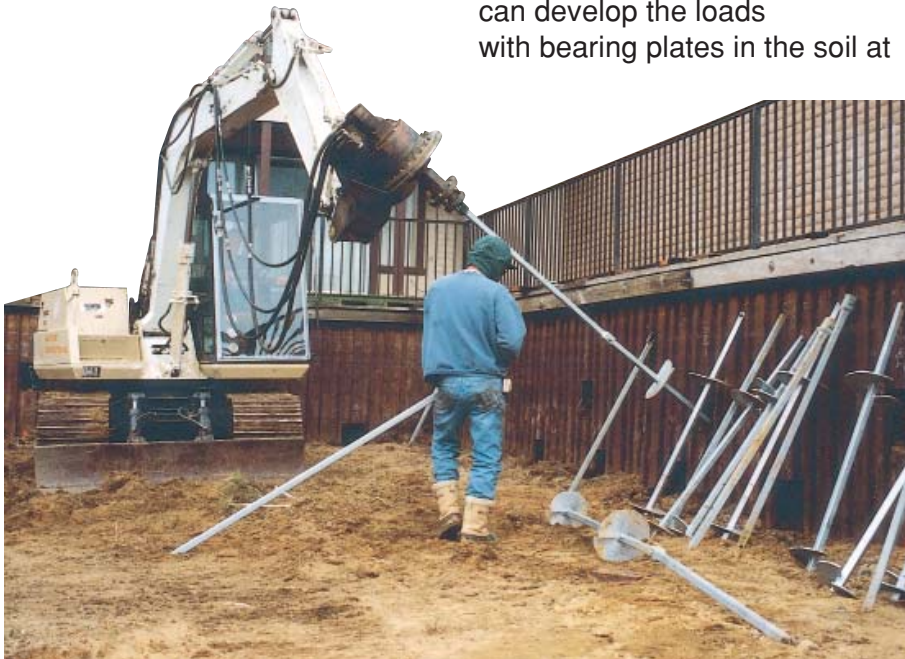
Track hoe makes maneuverability easy at lakeside sheetpile repair job.
