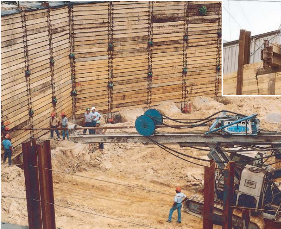
Lead-guided drill motors (crane-suspended or track-mounted) are common tieback drive equipment for large jobs.
