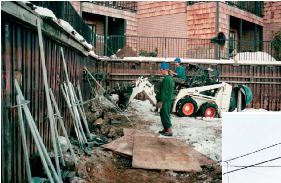
Skid-steer excavator powers Chance® hydraulic drive head mounted on special adapter plate.
