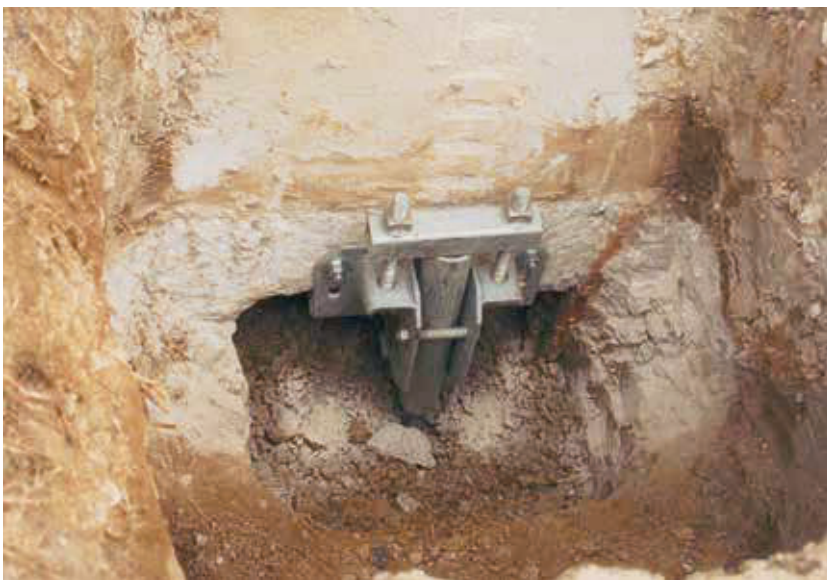
Completed helical pile and bracket
