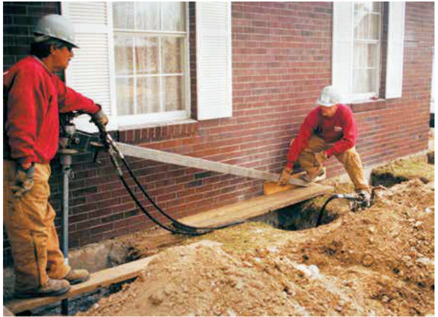
Helical pile installation by hydraulic driver
